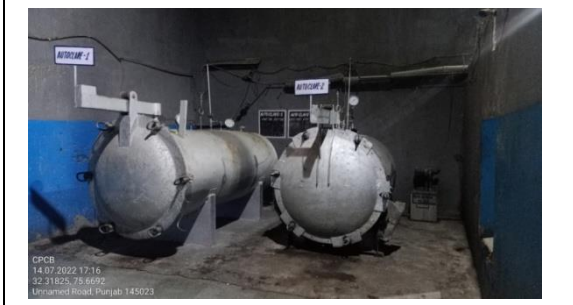
02 Autoclaves of total capacity 2850k/hrat CBWTF
